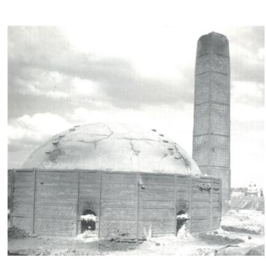
Figure 1: View of an igloo (or beehive) kiln and chimney
